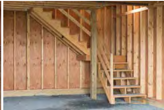
STEPS WITH LANDING AND HANDRAIL
